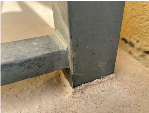
Railings embedded in concrete balconies
