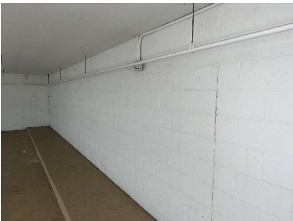
Paint finishes at garage
