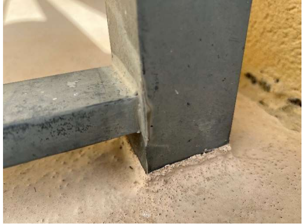
Railings embedded in concrete balconies
