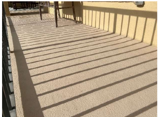
Concrete balcony overview
