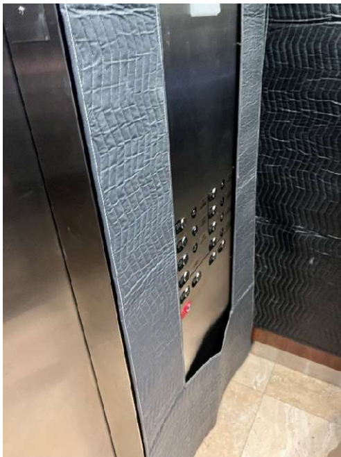
Elevator cab finishes
