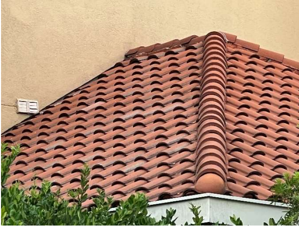
Lower concrete tile roof
