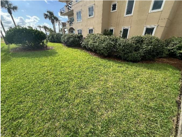
Area of below grade waterproofing
