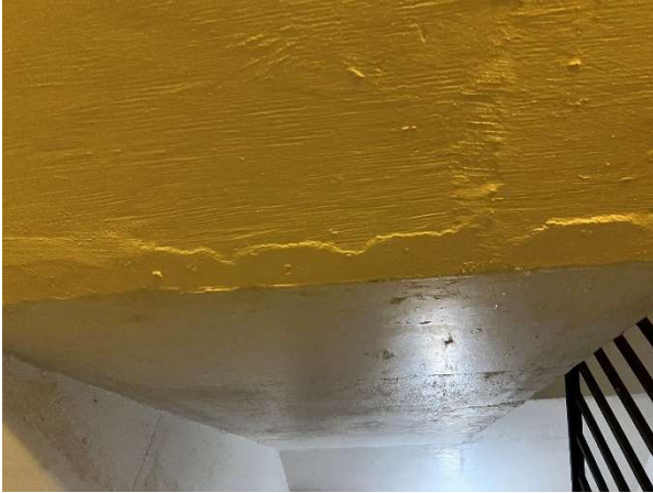
Detail view at finishes at stairwell
