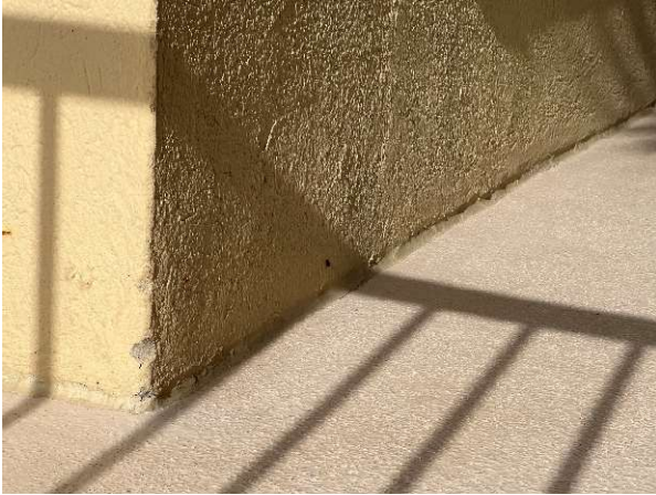
Concrete balcony joint to building
