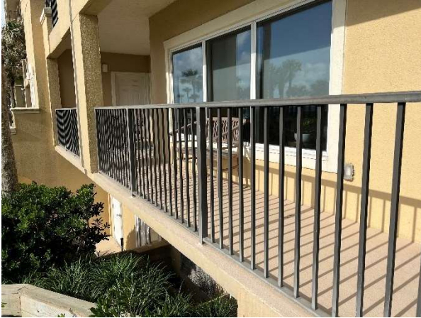
Balcony railing overview
