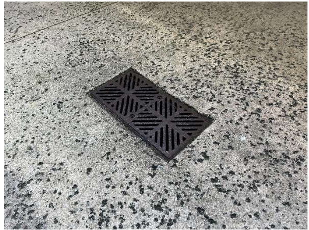
Concrete viewed at drain
