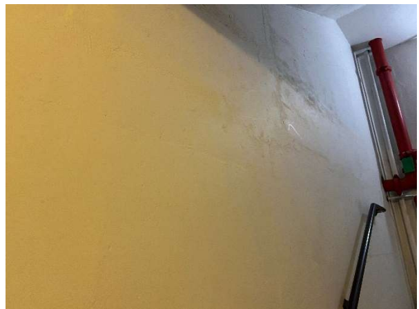
Wall viewed at stairwell
