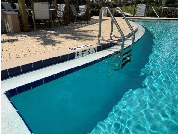
Pool plaster with tile at perimeter
