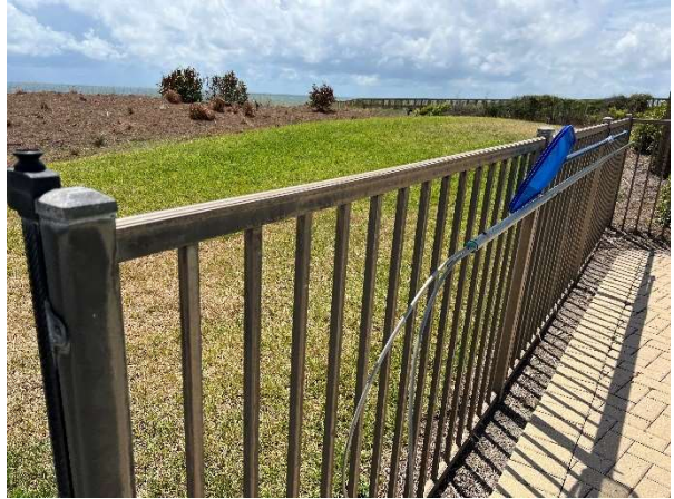
Finish deterioration
