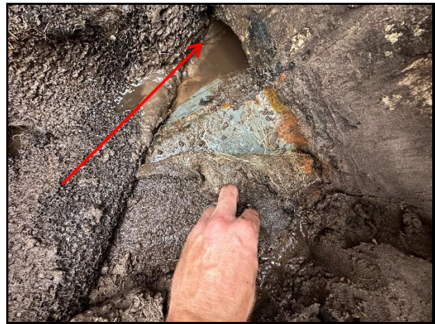
Photograph 26. Waterproofing with void through wall.
