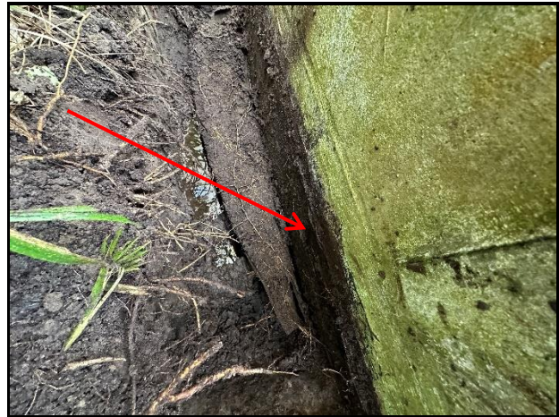
Photograph 30. Waterproofing is terminated below finish grade.
