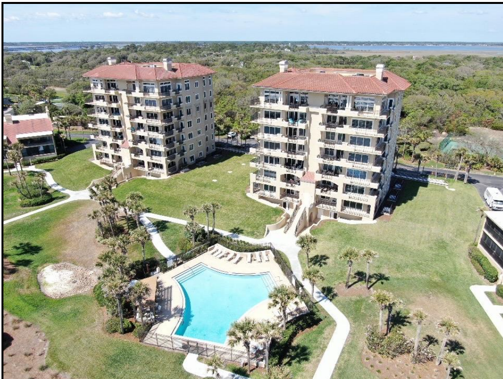
Photograph 10. Property overview – After construction.
