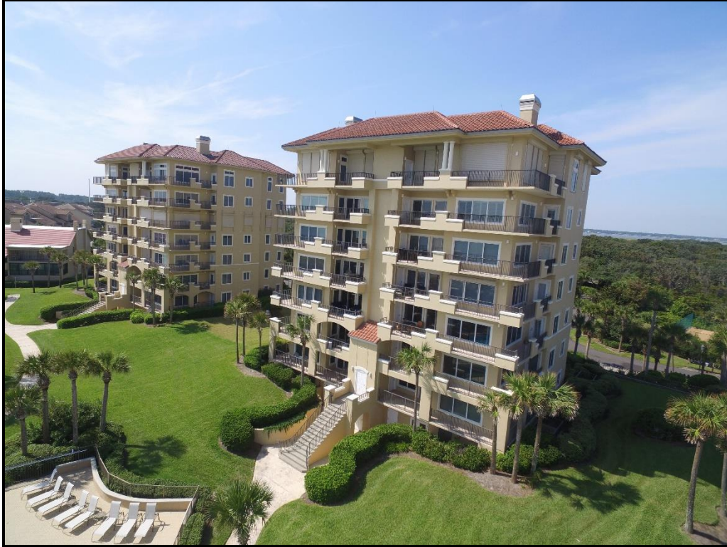
Photograph 5. Building 1 – Before construction.
