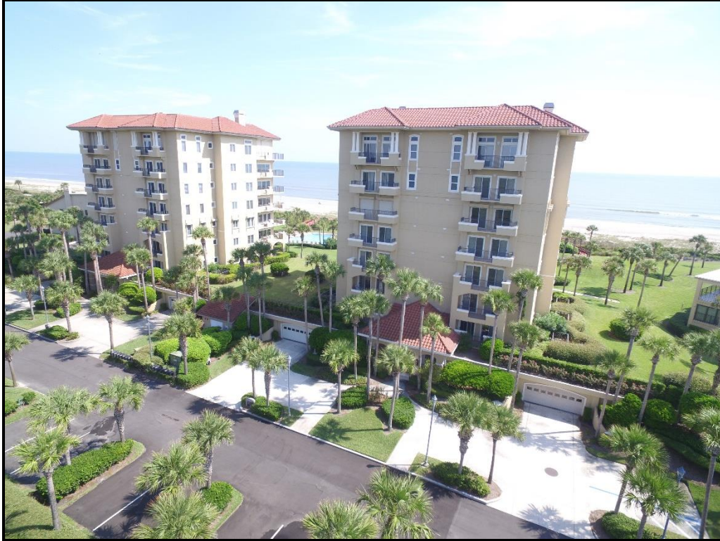
Photograph 3. Property overview – Before construction.
