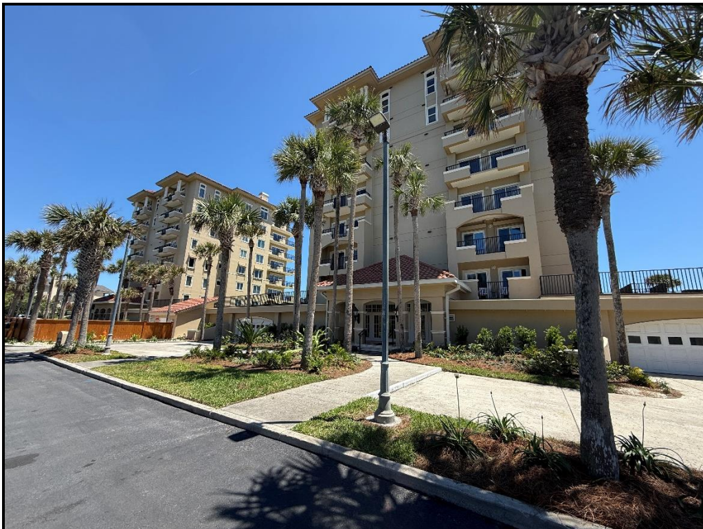
Photograph 8. Building 2 front overview – After construction.
