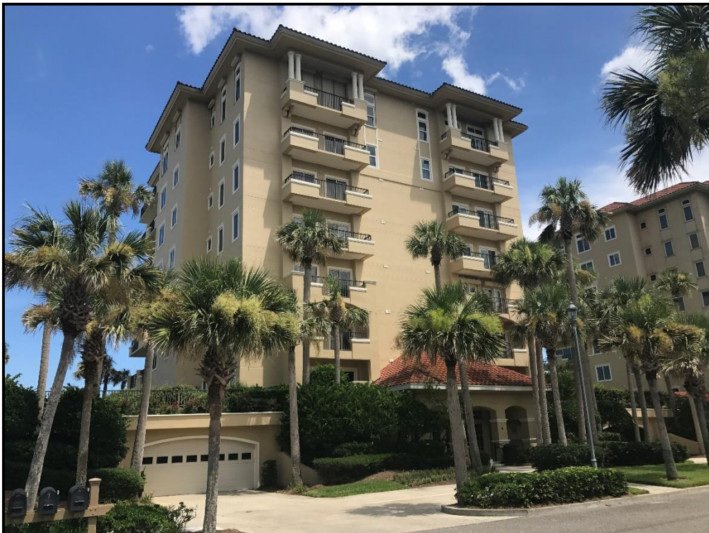
Photograph 2. Building 1 – Before construction.
