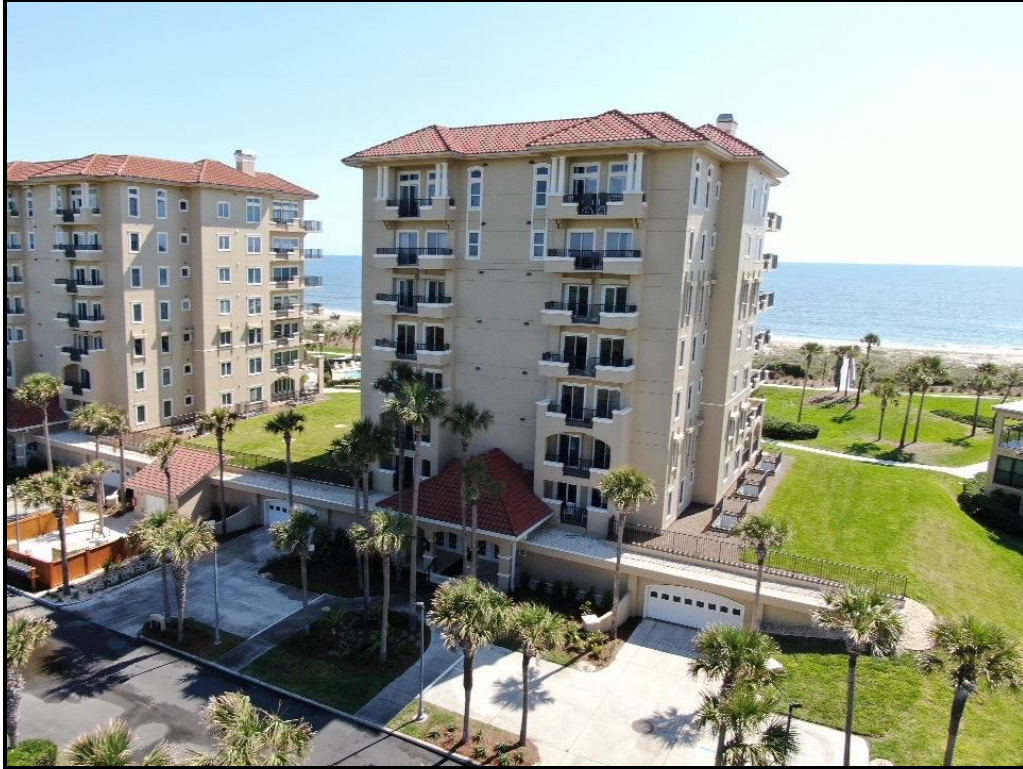
Photograph 7. Property overview – After construction.
