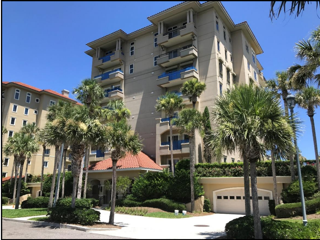
Photograph 1. Building 2 – Before construction.
