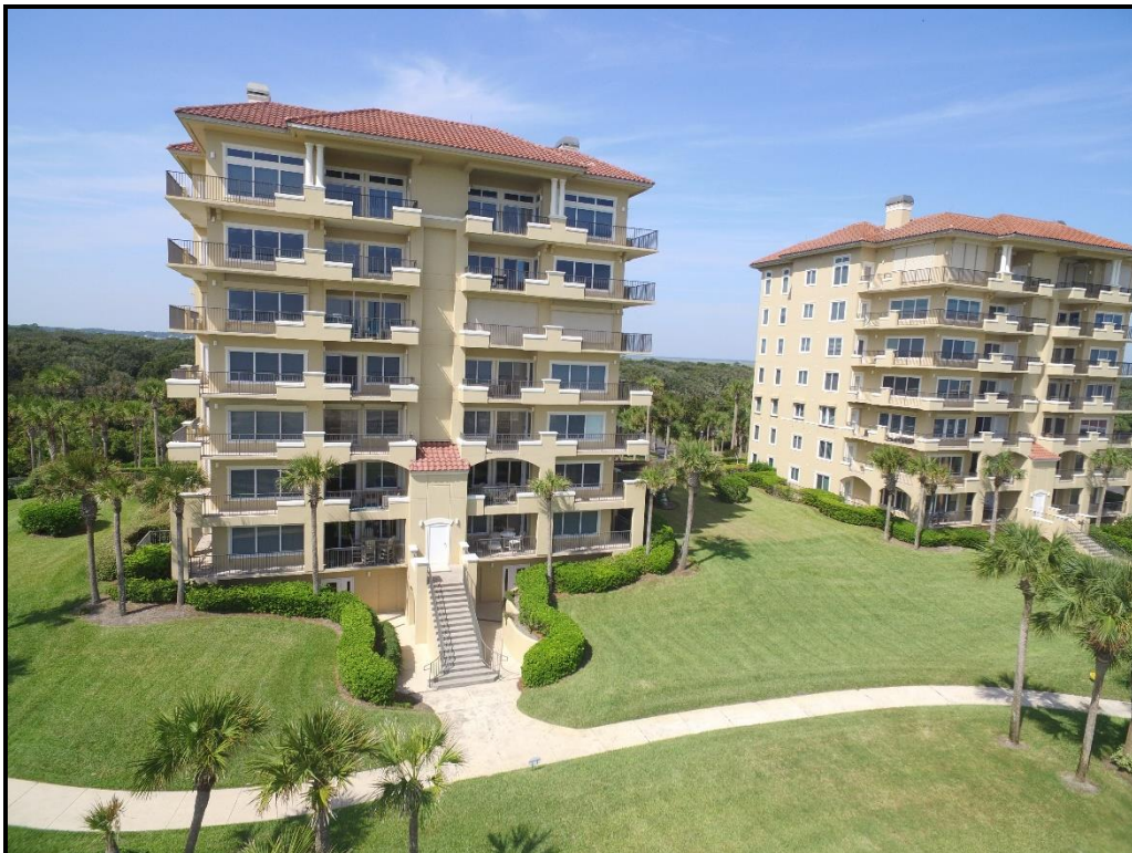
Photograph 4. Building 2 – Before construction.
