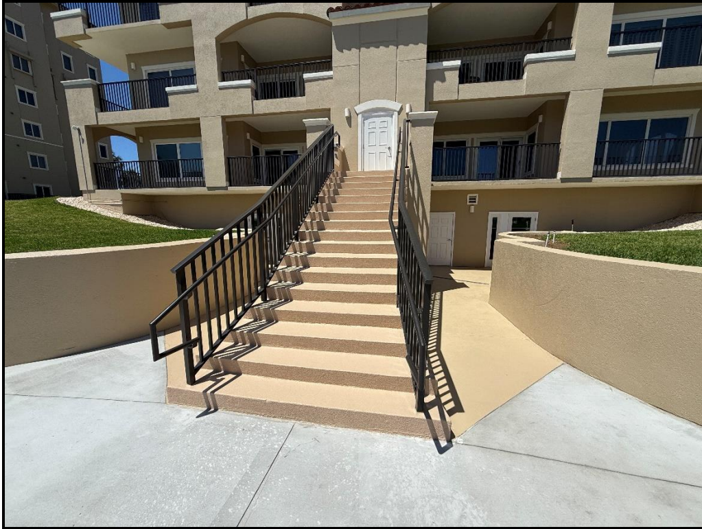
Photograph 9. East stairwell staircase – After construction.
